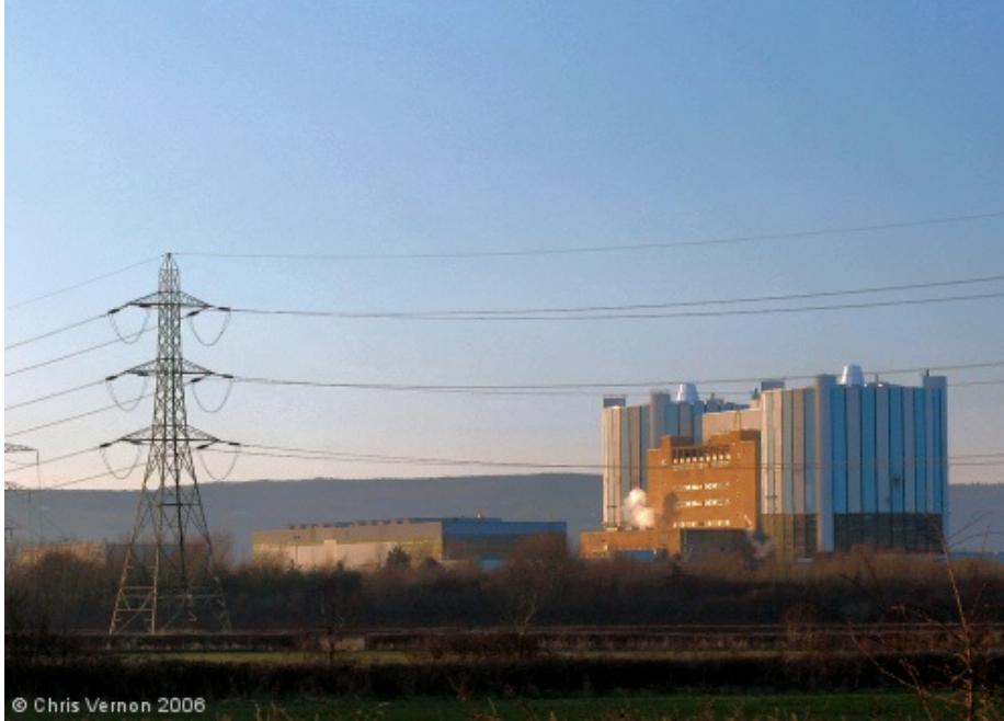
Oldbury Nuclear Power Station
