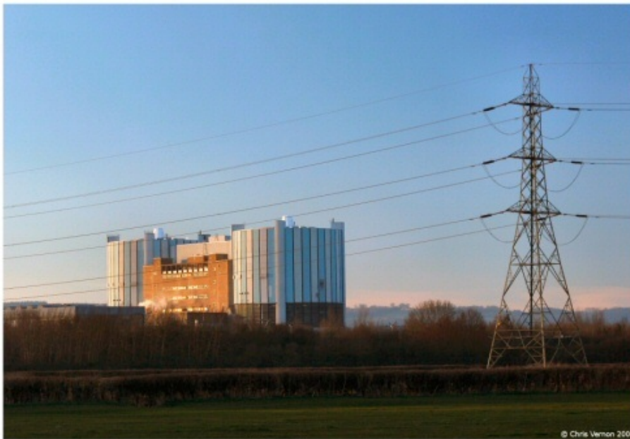
Oldbury Nuclear Power Station
